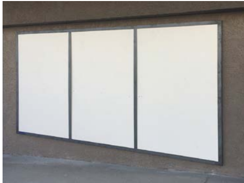
Blank panels shown installed with frame in place.
